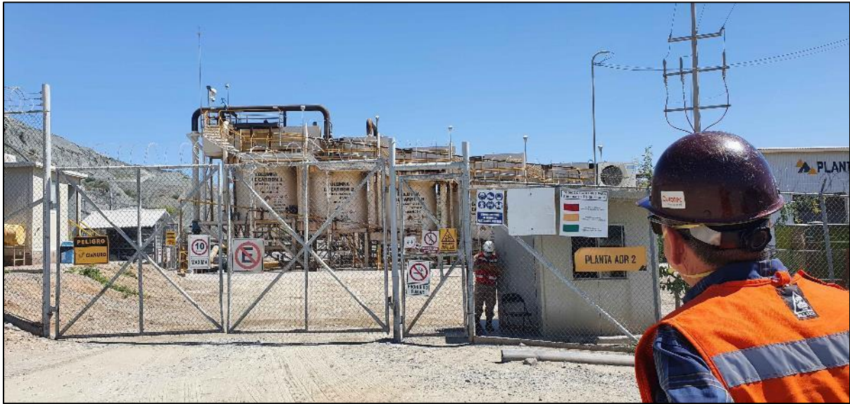
Figure 12.5 View of ADR Plant 2
