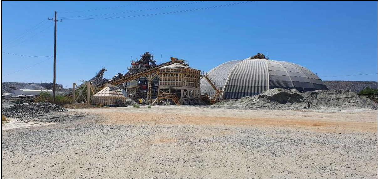
Figure 12.6 Partial View of the Crushing Facility
