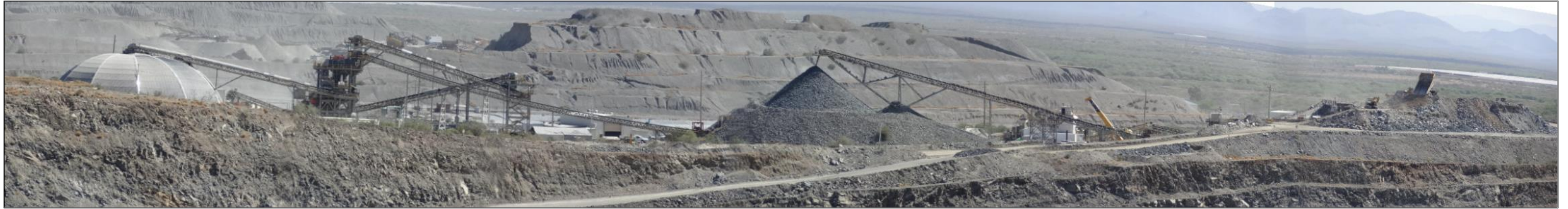
Figure 17.7 View of the Crushing Facilities and Heap Leach Pads as Seen from the Lookout at the San Francisco Pit (Zoom Lens)
